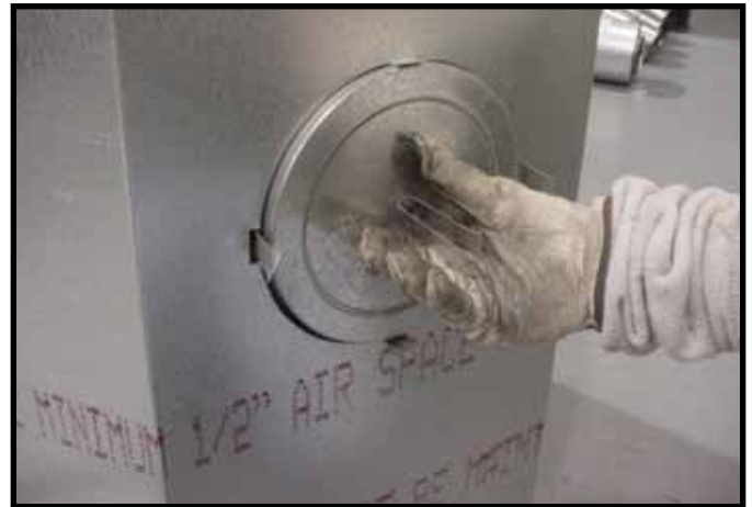
Figure 9.9 Fold the center parts of the retaining band out and use to remove the seal cap.
